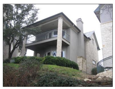
5551 likely applies. While under the roof line, this balcony projects from the building exterior surface and is supported by columns. Expect the rock on the column is just veneer over wood structure.
