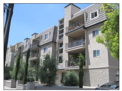
5551 likely applies. While the bulk of the balcony is within the exterior profile of the building, there is a projected portion and leaning against the railing is potentially hazardous.
